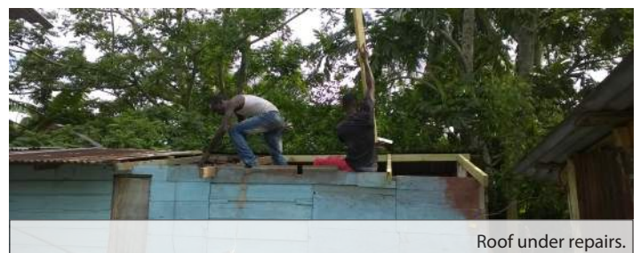
Retrofitting underway in earnest.
