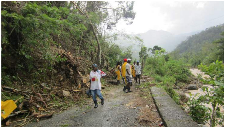
Flood rains damage infrastructure and farm lands in eastern Jamaica.
