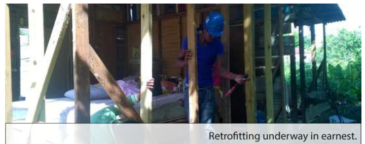
Rotting boards in St. Thomas dwelling.
