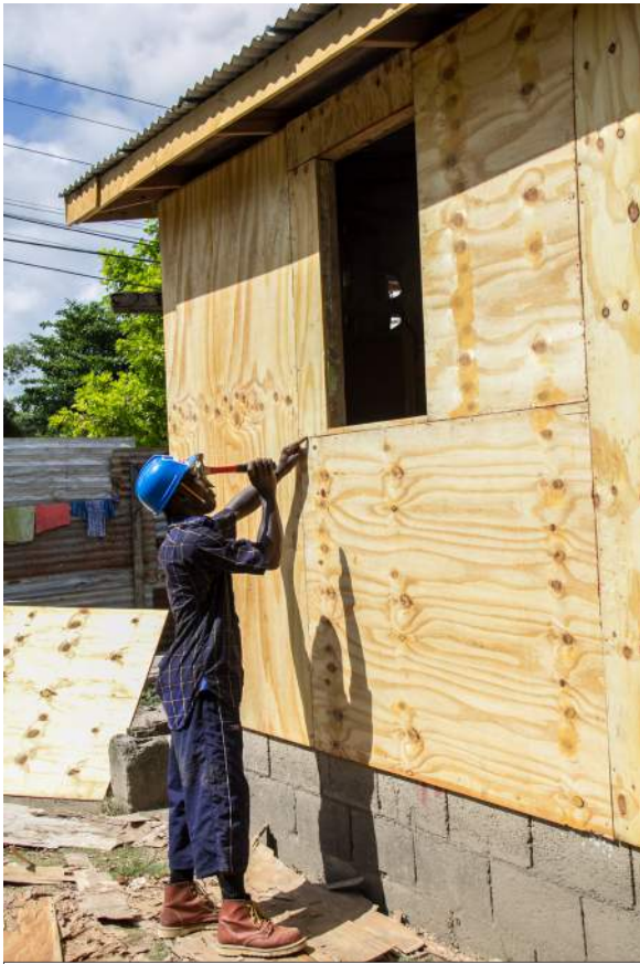
Volunteer assists in the retrofitting exercise in St. Thomas.
